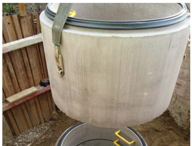
Large ring lowered into position
