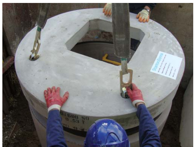
Lowering slab to complete manhole section
