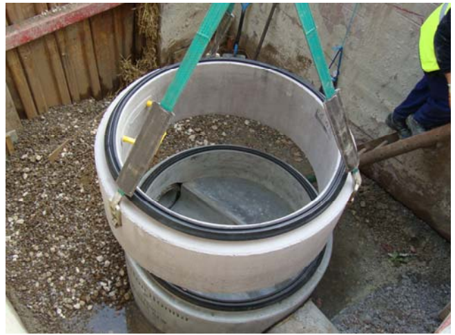
Once base secured and level ring is lowered into place
