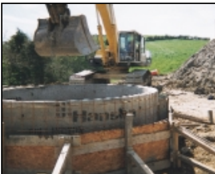
4 metre manhole under construction
